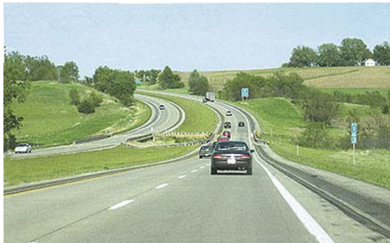
SAFETEA-LU contains changes in funding and other areas to meet the challenges of maintaining and growing transportation infrastructure such as the highway shown here.
